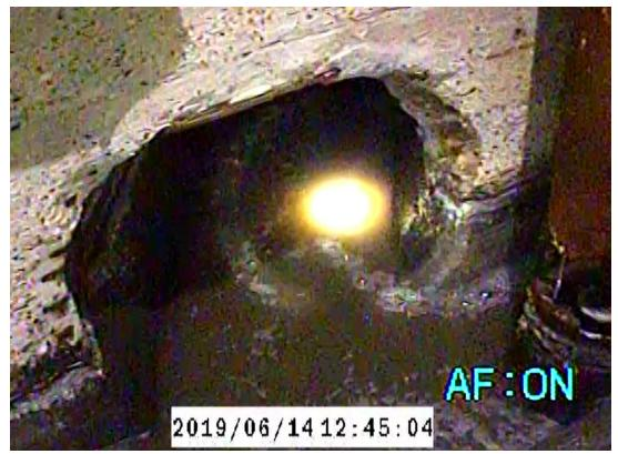
West Wet Well showing 1500mm Diameter Inlet Wastewater Pipe
