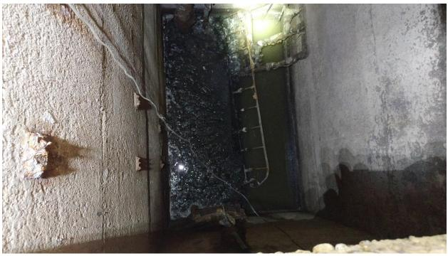
East Wet Well with Fallen Ladder Section
