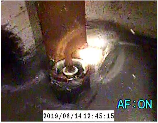
West Wet Well Showing Storm Pump Suction Pipe
