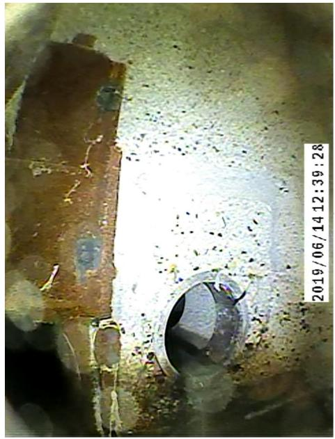
West Wet Well Looking at 600mm Diameter Inlet and 375mm Diameter Inlet Wastewater Pipes
