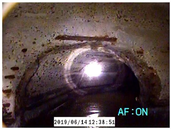
West Wet Well Looking Down 1500mm Diameter Inlet Wastewater Pipe
