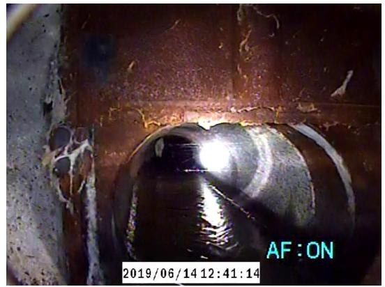
West Wet Well Looking Down 600mm Diameter Inlet Wastewater Pipe
